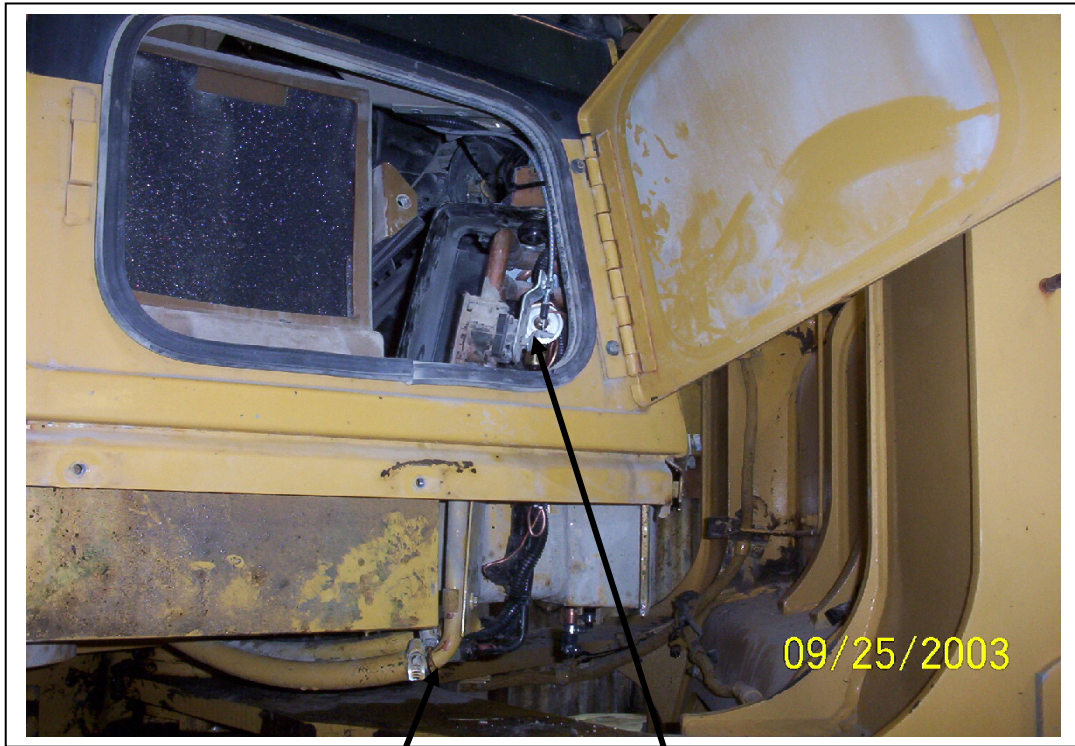
A/C hoses connected to the A/C pipes.
